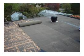
Fig. 2. Moisture proofing using bitumen
