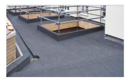
Fig. 3. Moisture proofing using asphalt
