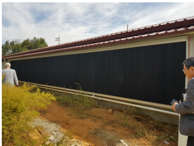
Figure 5. Seawater curtain to suppress AIV in aeolian dusts.
