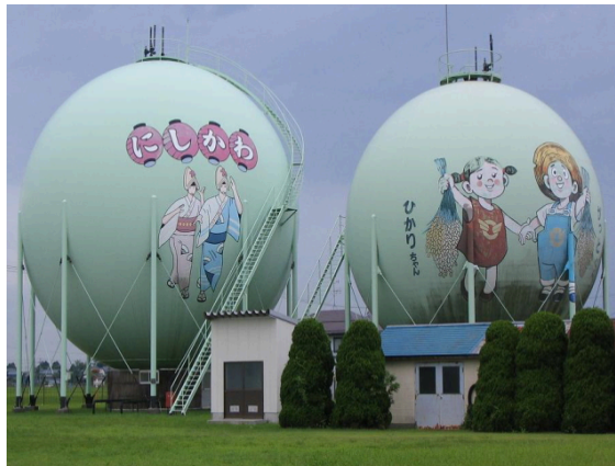
Figure 1. Japanese gas companies added a touch of character to giant spherical gas tanks.
