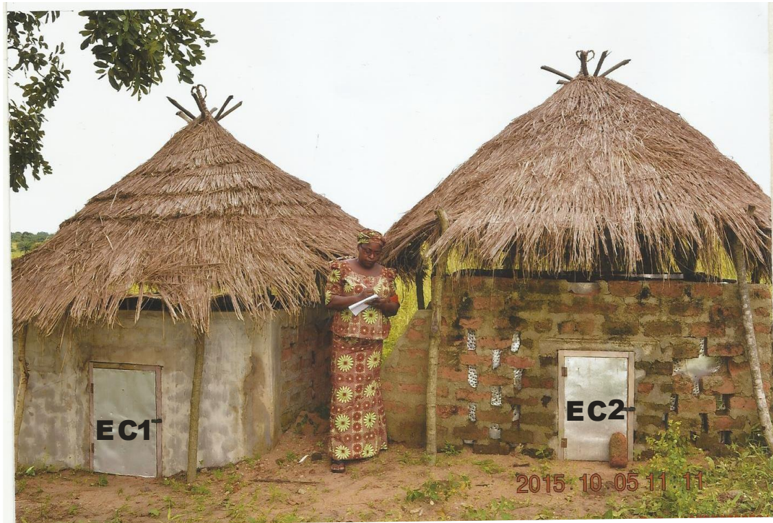
Plate 1. Evaporative coolers 1 and 2. EC1= Non-Cladded Burnt-clay-brick evaporative cooler (NBBEC) EC2= Aluminum-Cladded Burnt-clay-brick evaporative cooler (ABBEC)
