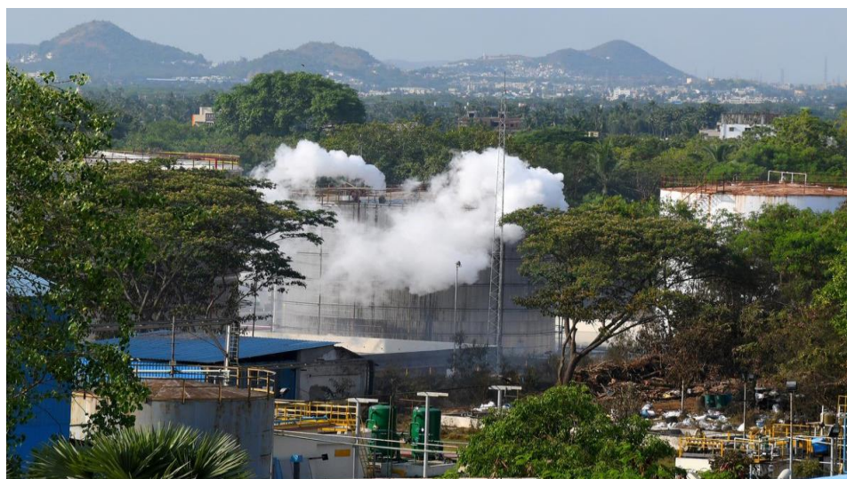
Fig. 3. A file photo of styrene gas leaking out of a tank in LG Polymers unit, in Visakhapatnam
