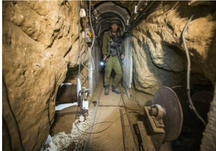
Figure 4. Tunnel with electrical. Reprinted with permission from Editor of Open Journal of Soil Science.
