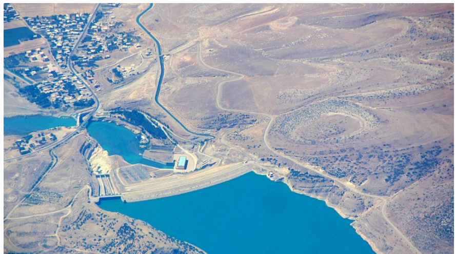
Figure 6. Batman Dam in Türkiye. Photo credit: Rehman Abubakr.
