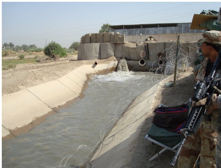
Figure 28. The secured Yusifiyah Pump Station #2 and feeder canal supplies water from the Tigris River. Photo credit: David R. Speidel, U.S. Department of Agriculture.
