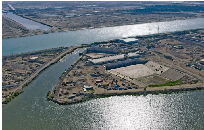
Figure 20. Nasiriyah Drainage Pump Station. Photo credit: special inspector general for Iraq reconstruction.
