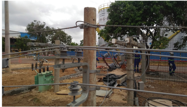
Figure 6. Deflection structure from 7° to 45°.
