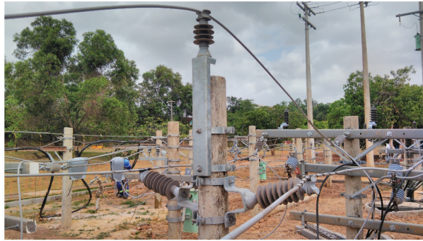
Figure 3. Utility structure with wooden pole.
