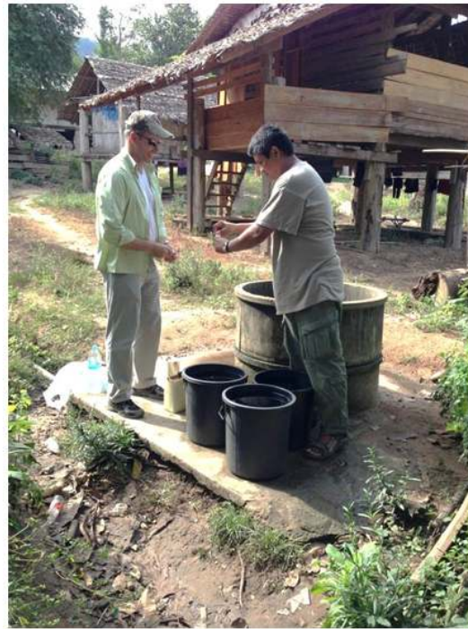
Fig. 2. Sampling wells in the village. Note the concrete apron base is exposed. Well rings were fully cemented, but no wells had covers
