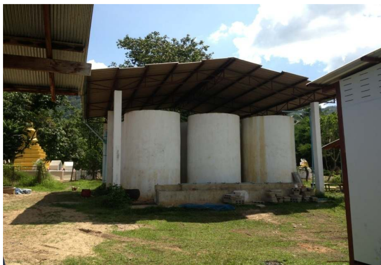
Fig. 9. Existing rainwater harvesting system for the village school
